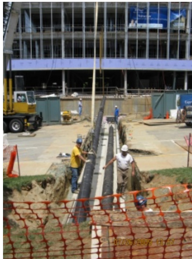
Figure 4: Steam tunnel entering south side of building.
