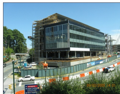
Figure 2: South West Façade
