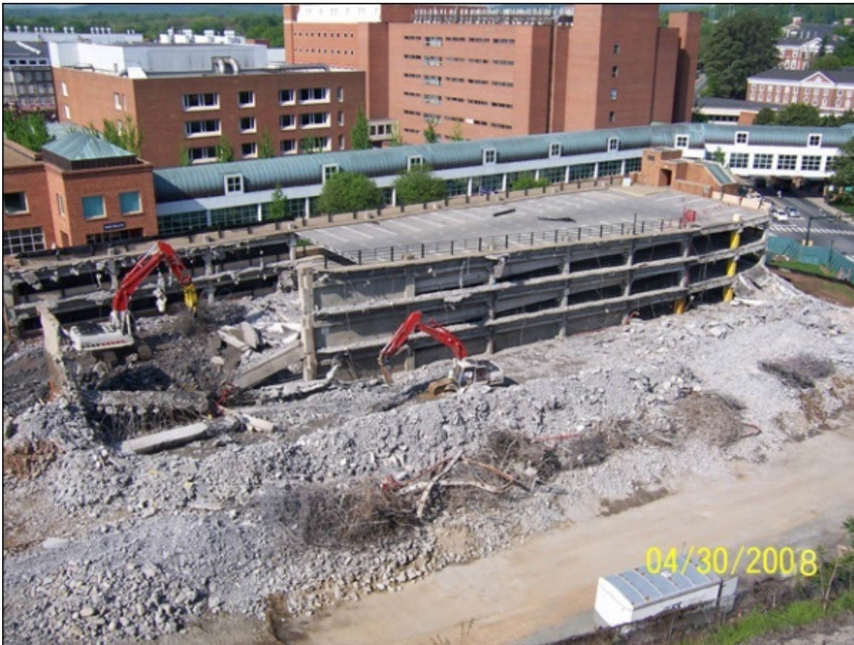
Figure 6: Garage demolition. Picture provided by The University of Virginia.
