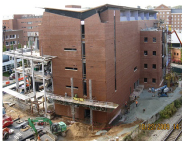
Figure 1: North East Façade
