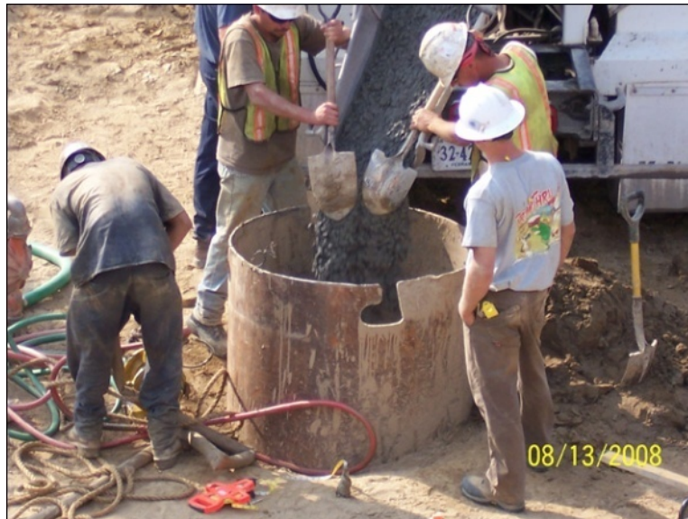
Figure 5: Caissons being placed. Picture provided by The University of Virginia.
